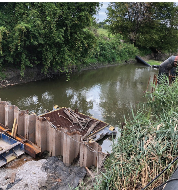
Sheet piling and dam construction prior to slipline rehabilitation.
