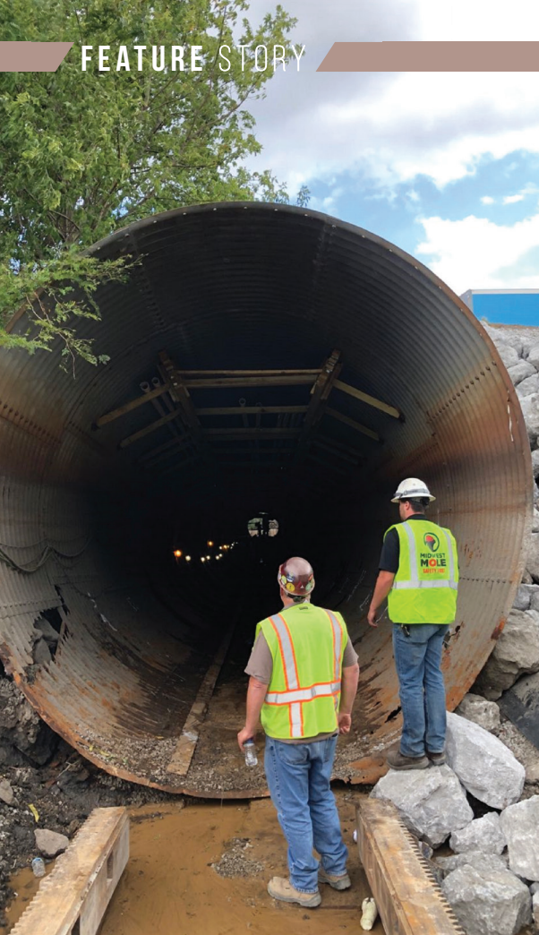
Existing culvert condition prior to rehabilitation.
