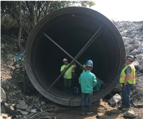
Reducing section, located on upstream end of culvert.
