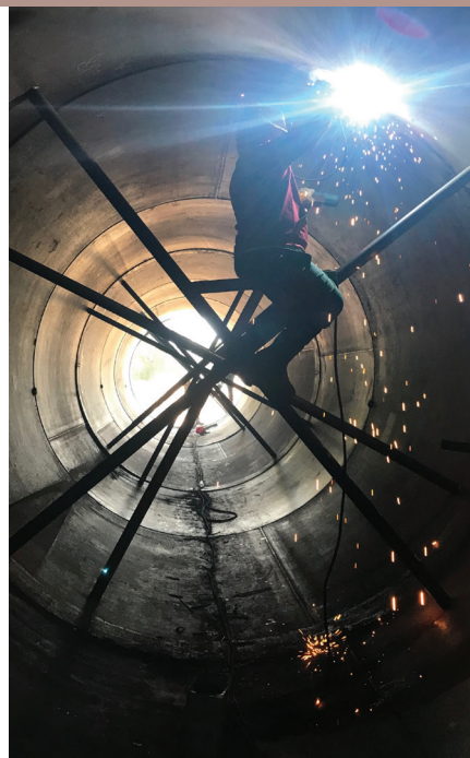
A welder works in the interior of the liner to join liner sections. The full penetration welds limit the possibility of joint failure.
