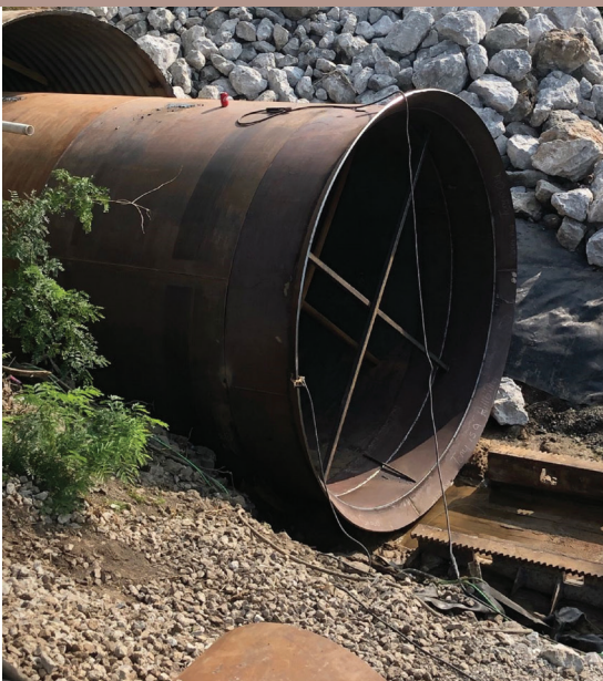
Reducing section, located on upstream end of culvert.
