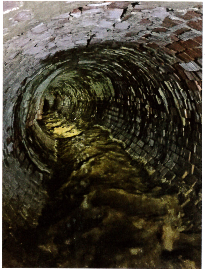
ORIGINAL BRICK SEWER SHOWING CURVED SECTION.
