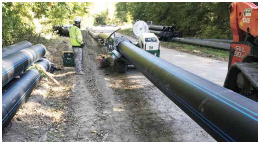
Under the river segment was fused all in one long run
